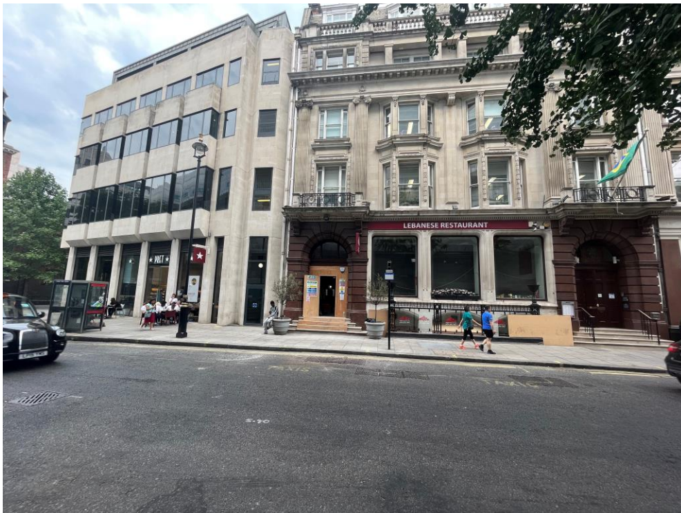
View of 3-4 Vere Street and 1 Chapel Place from the west side of Vere Street
