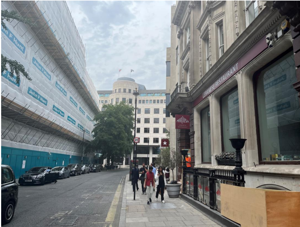
Vere Street looking north, 3-4 Vere Street on right hand side
